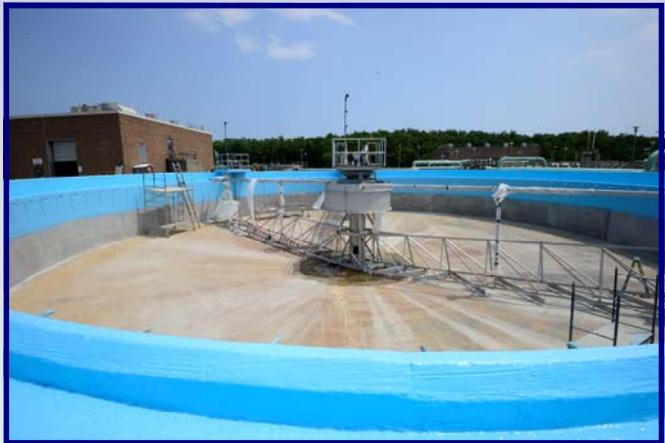
Not to be outdone, the central plant started demolition of PC-2 during the latter part of April with the final segment of the work completed by mid-May. This allowed Aulffo Painting to begin the arduous task of removing the existing coating system at PC-2. Once finished, Stone Hill proceeded with the installation of the new coating and finalized the installation of the new mechanical system by the end of July with startup scheduled during the first week of August.
