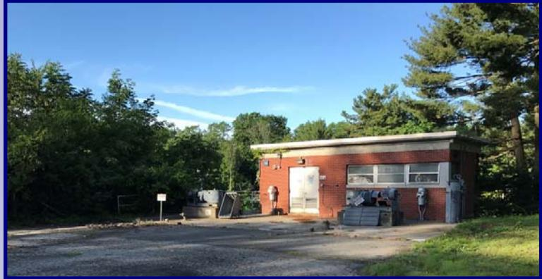
Beginning in early August, demolition of the existing carbon building will take place. Testing was conducted to confirm the absence of asbestos in the roofing material of the carbon building, and the tests showed no signs of asbestos. Currently the interior fixtures are being removed, and demolition of
