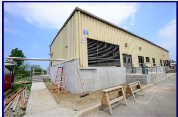
Hays Sheet Metal has started installing the new louvers in the blower building. Stone Hill has completed installing the new PS Doors flood gates in the combined blower building. The new Neuros Turbo Blower is scheduled to be delivered at the end of August.
