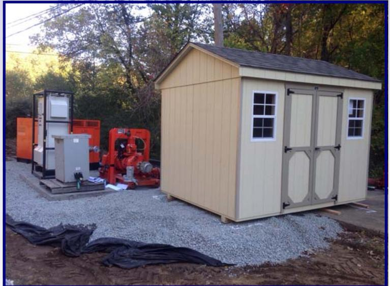
The existing structure was then demolished while protecting the existing pumps and piping that were left in place for reuse. Work continued with a masonry knee wall and framing for the new building, siding, roofing, and doors and windows. All new electrical work, plumbing and mechanical upgrades were then installed to bring the pump station back to full use.
