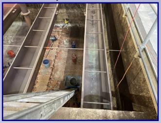
After the media was reinstalled, the complete system was then backwashed and core samples taken for conformity. The filter was then chlorinated and at press time is going thru several backwashes and sampling for arsenic and coliform. Once a sampling provides levels of acceptance, the filter will then be put online, and Stone Hill will proceeded to the next filter.
