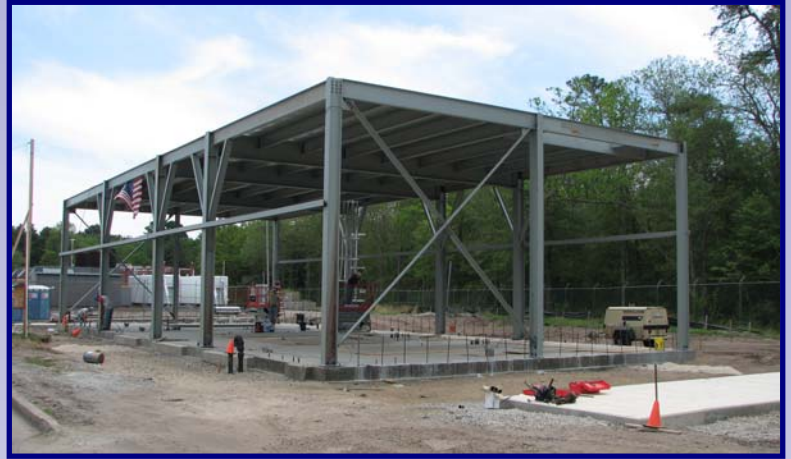
Structural Steel at the Emergency Generator Building
