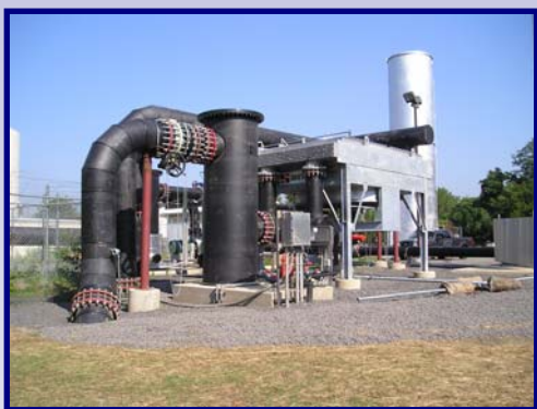
New Unrestricted Gas Bypass Lines and Aftercooler Installation
