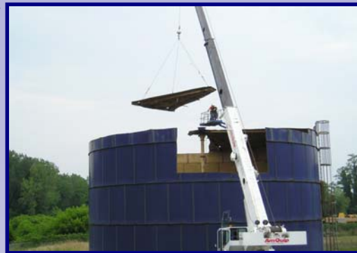
Demolition Begins on the 500,000 gal Storage Tank
